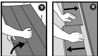
**11.** Separate the whole row by carefully lifting up and slightly knocking just above the joint. Fold up and release the whole side.
